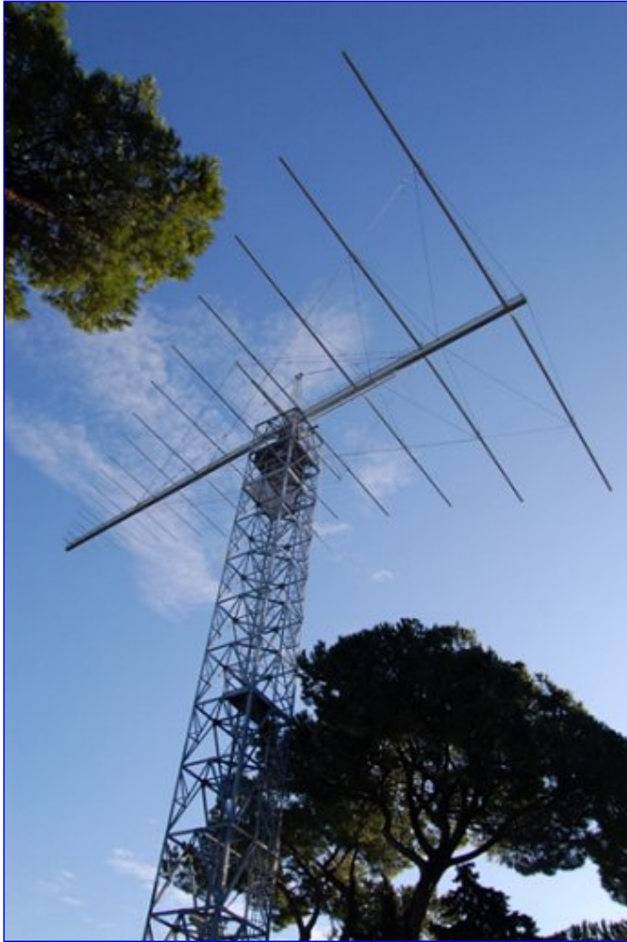
H.F. Log Periodic on Tower.
